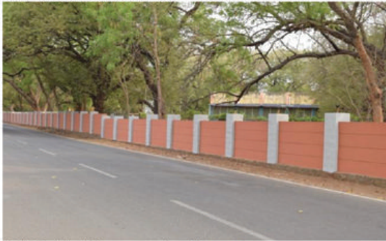
Well Painted Compound wall
