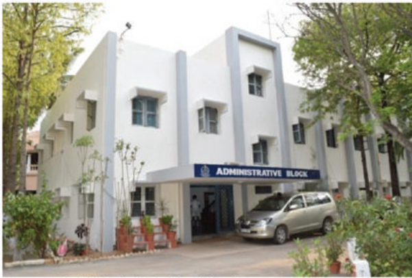
Renovated Administrative block
