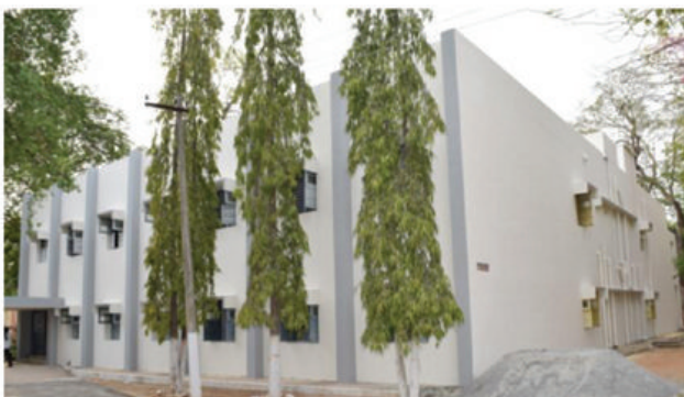
Renovated Trainee officers' hostel
